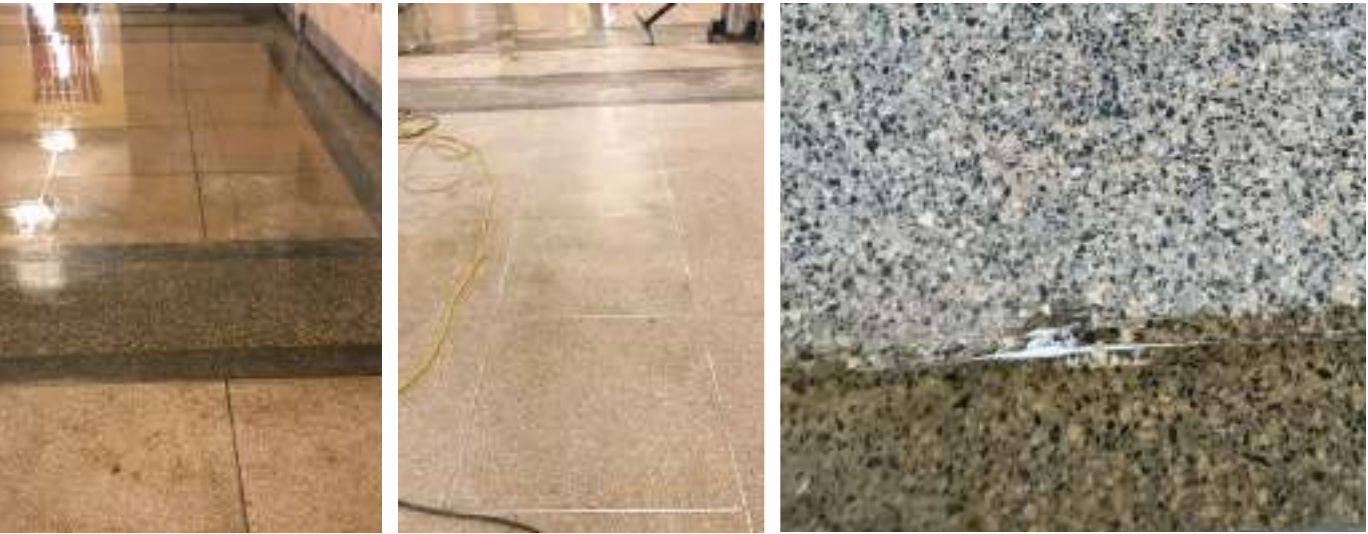
Photos, from right: Floor with 50 years of wax buildup, Stripping off the many layers, and Close-up of wax on and wax off.
